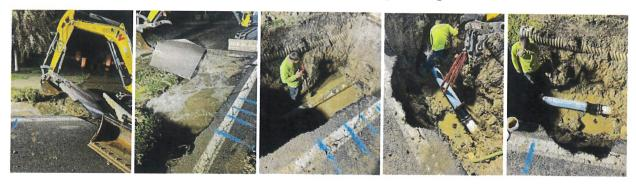
• Smith Corp has completed the installation of the main waterline and stormwater line, including the manholes. They are currently working on the lateral lines. Once this work is finished, they will schedule the repaving of the street. The project remains on track to be completed in May.
